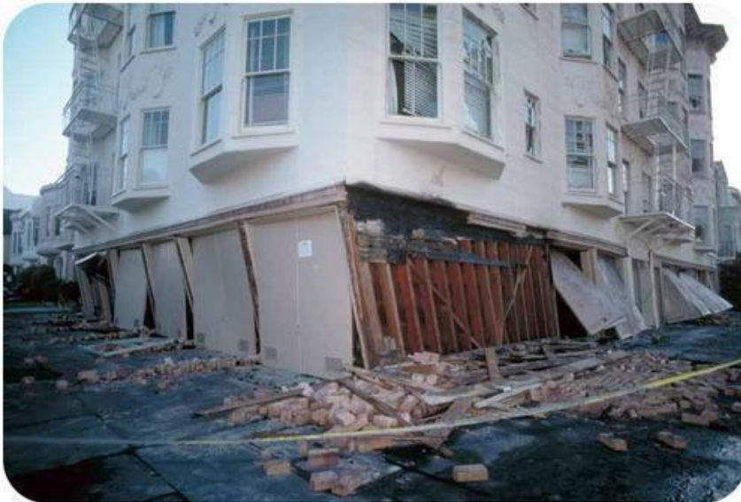
In this image, the first floor of this San Francisco building is collapsing after the 1989 Loma Prieta earthquake
