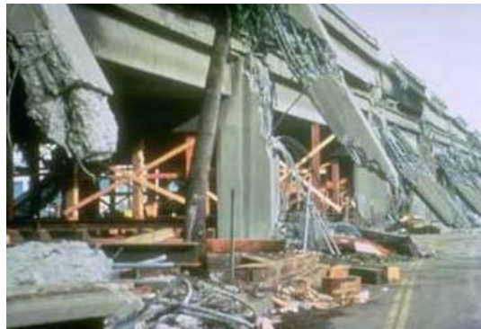
Figure 4.28 Collapsed bridges – USGS
